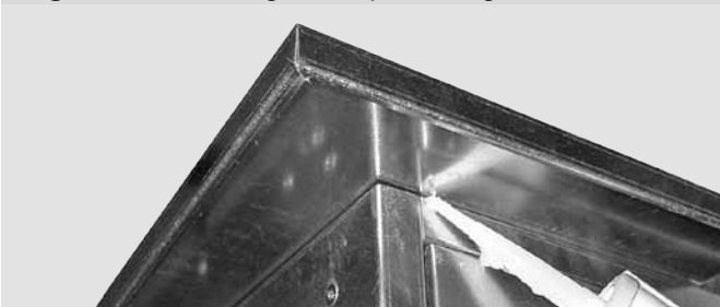
Figure 14 – Sealing of the panel edges
