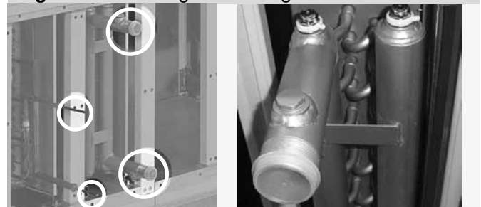
Figure 17 – Heating and cooling media feed
