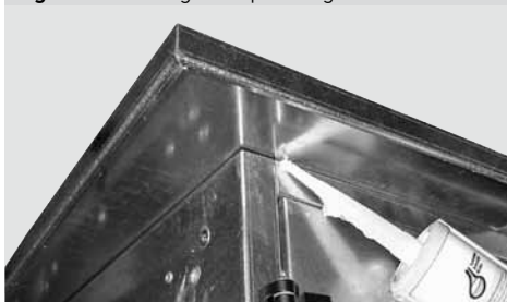
Figure 13 – Sealing of the panel edges
