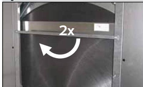
Figure 2 – Rotor Fixation Removal
