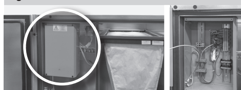
Figure 13 – switchbox
