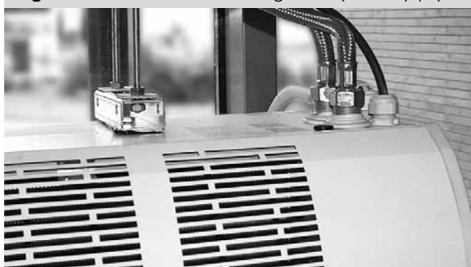
Figure 13 - connection of heating water (flexible pipe)
