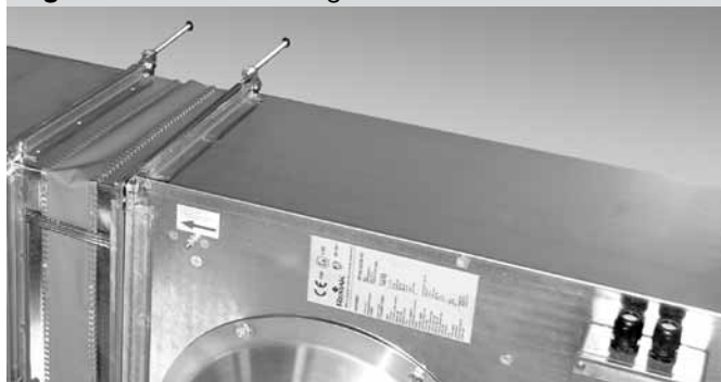
Figure 13 – Fan anchoring
