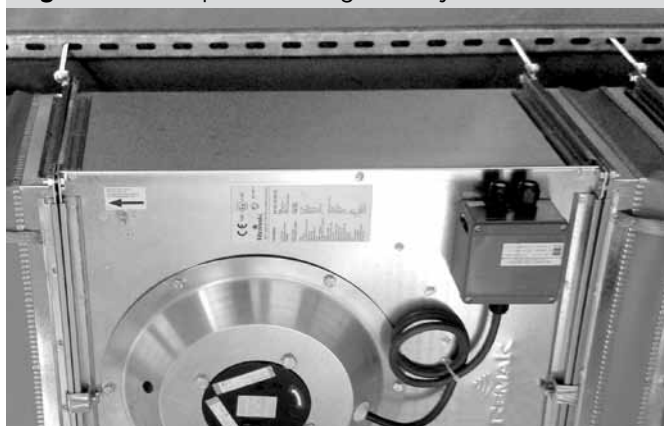
Figure 14 – Suspension using ancillary construction
