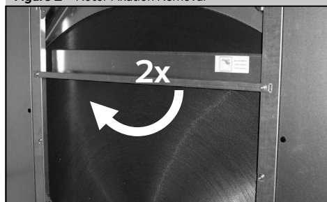
Figure 2 – Rotor Fixation Removal
