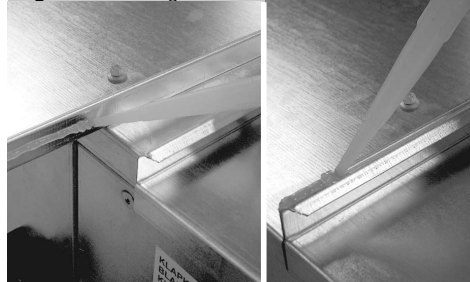
Figure 10 – Sealing of roof elements
