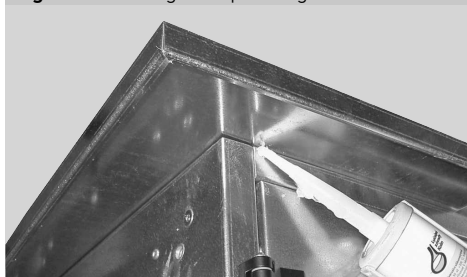
Figure 13 – Sealing of the panel edges
