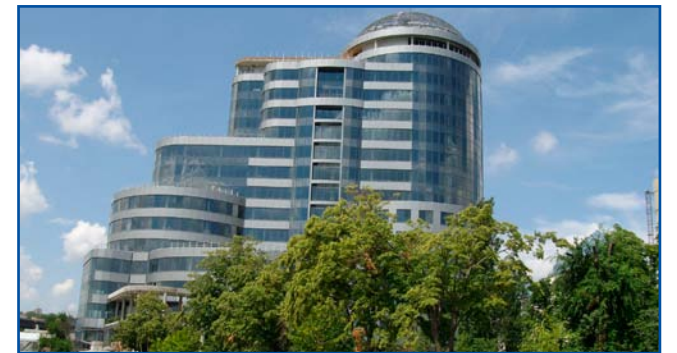
ADMINISTRATION CENTRE Rostov-on-Don, Russia
